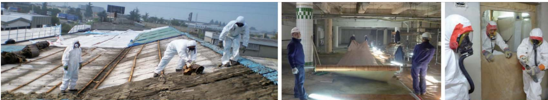
SERVICE: Removal of asbestos and MMVFs
